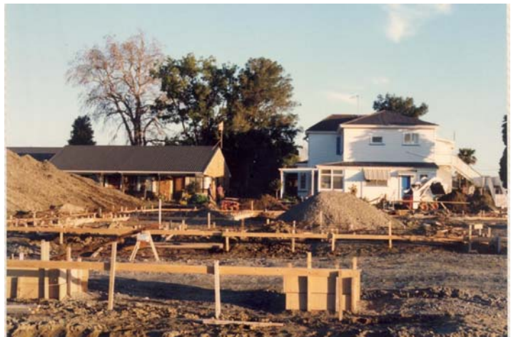
Early stages of Taradale site
